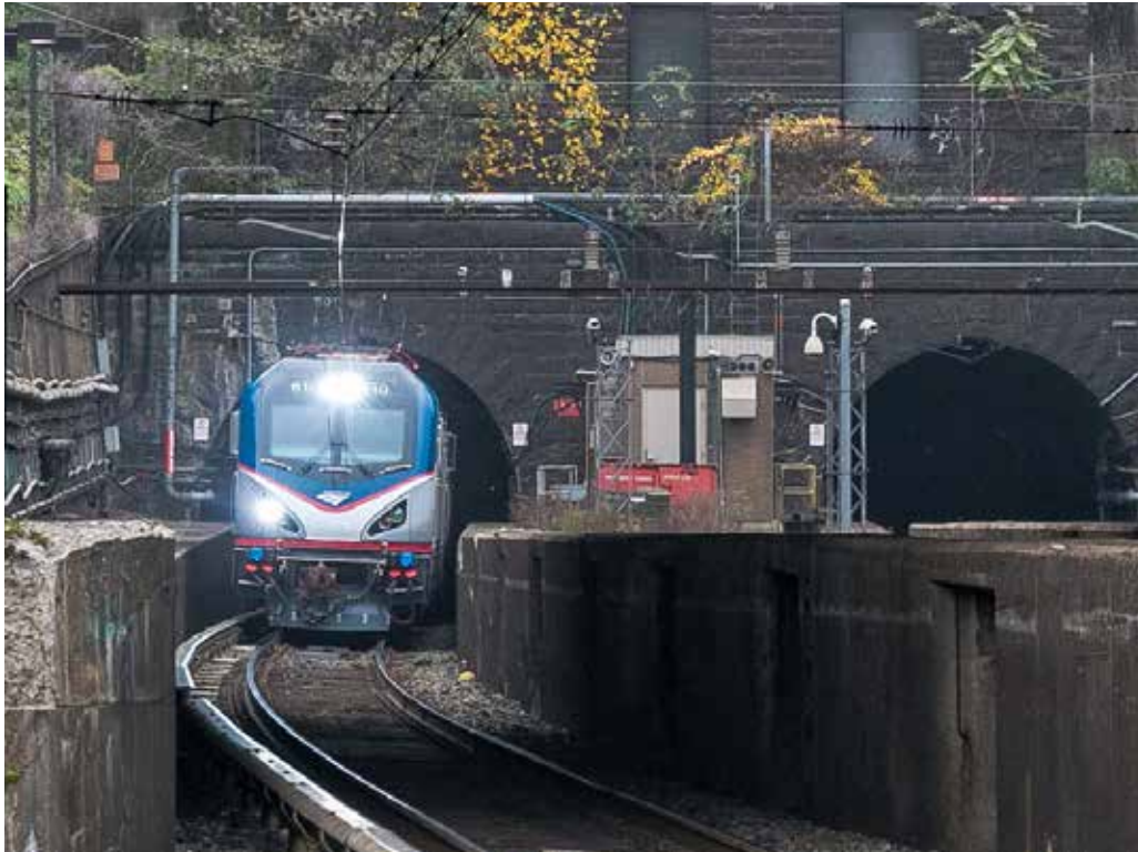
At left: Weehawken Portal of the North River Tunnel. Opened in 1910, the existing two-track North River Tunnel carries passengers between Manhattan and New Jersey underneath the Hudson River.
